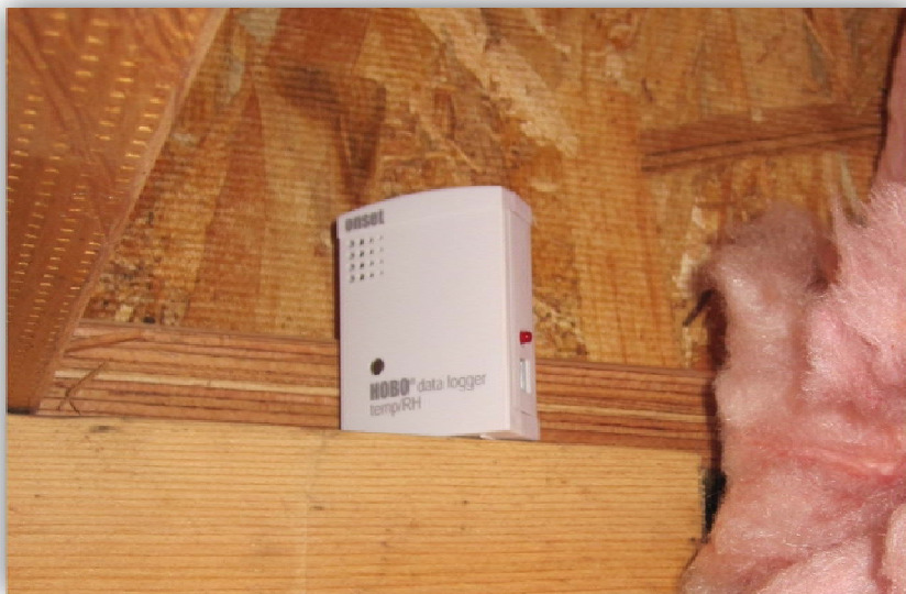
Figure 4. Integrated temperature loggers were installed in each crawlspace.
