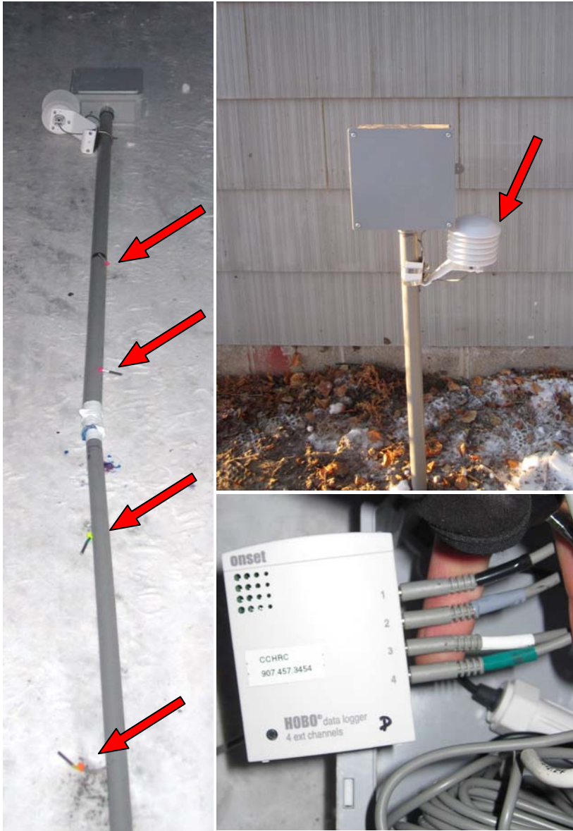
Figure 9. (Clockwise; starting from left) The probe assembly prior to installation; the assembly after installation; one of the two data loggers contained within the housing. The soil temperature probe assembly housed the temperature sensors and data loggers.
