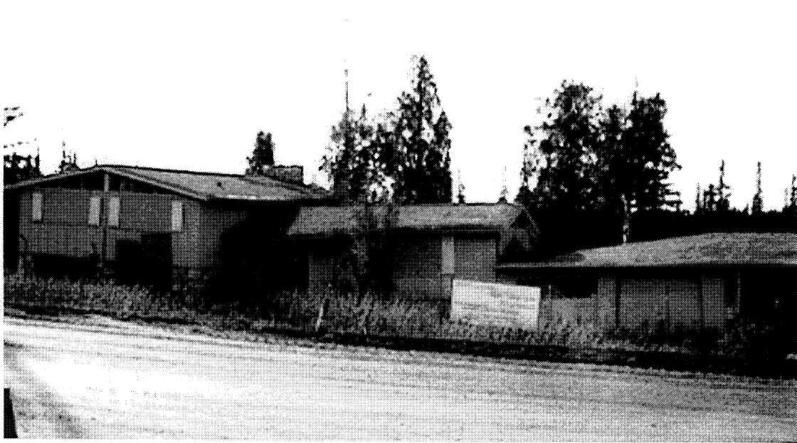
Figure 1.6 A house built in Fairbanks, AK on thaw unstable permafrost. This house with its heated basement eventually deteriorated until it was uninhabitable. It was finally burned because it had become a safety hazard to the community.
