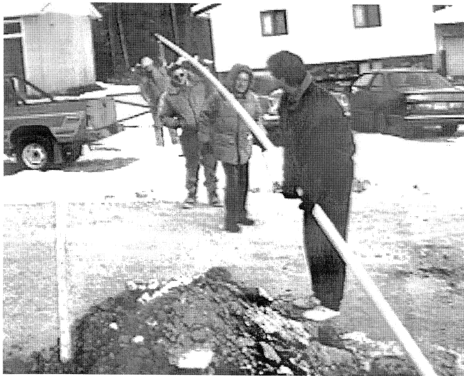
Figure 5.9 Feeding the thermosyphon pipe back into the hole attached to the drill stem as the drill stem is withdrawn.
