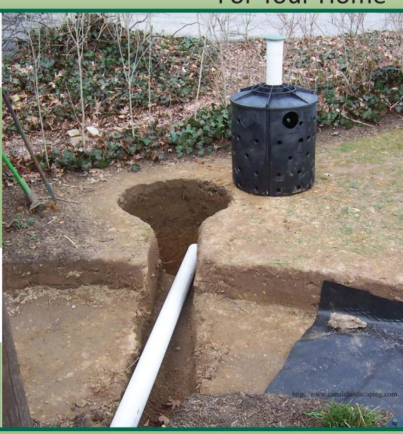
A dry well is a perforated pipe that drains into a small pit filled with gravel. Only roof runoff should be redirected into a dry well. The following instructions are for a very simple dry well. If your yard frequently floods you may want to install more than one dry well.
