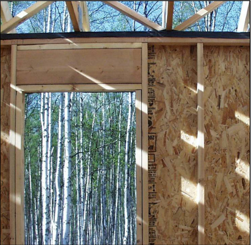
Image 23. Strip lapped over top plate and sealed to interior ceiling vapor retarder and exterior membrane
