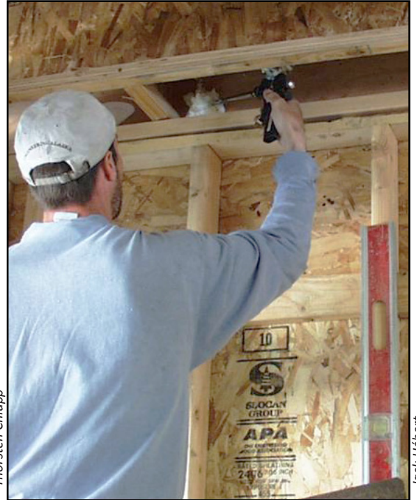
Image 4. Insulating deck fastener penetrations on interior to prevent condensation
