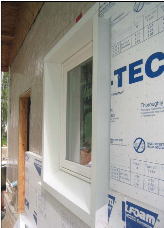
Image 15. Inset window with steel jamb extension
