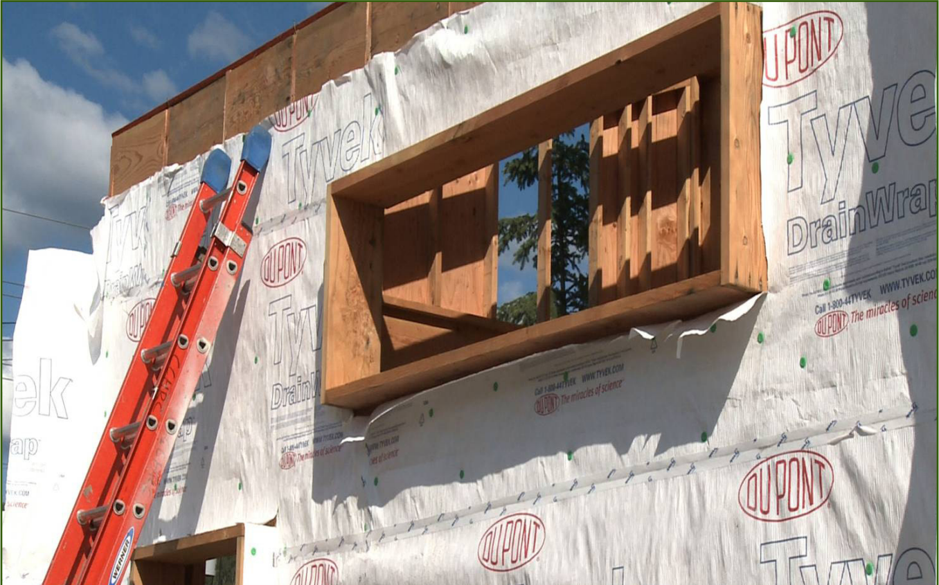
Image 21. An exterior air barrier is optional and subject to codes
