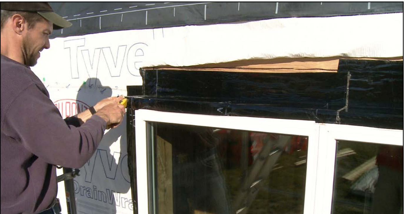
Image 11. Shingle-style flashing on exterior window buck
