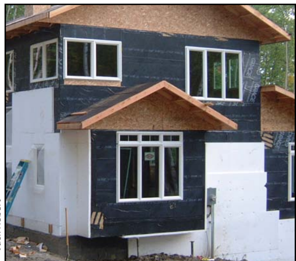
Image 29. Cantilevered addition wrapped with foam board
