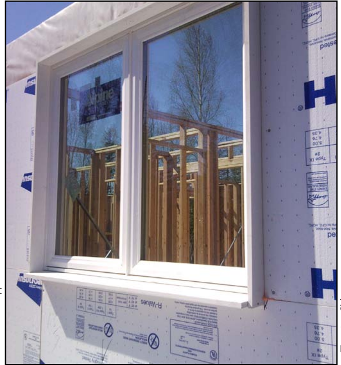
Image 14. Inset window with AZEK® and first layer of foam
