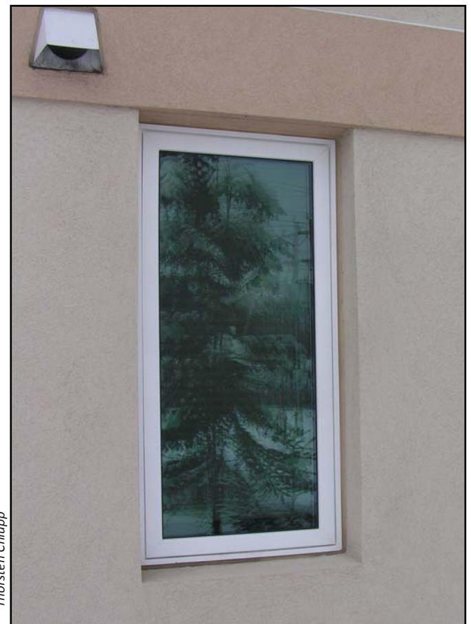
Image 16. Inset window with stucco exterior
