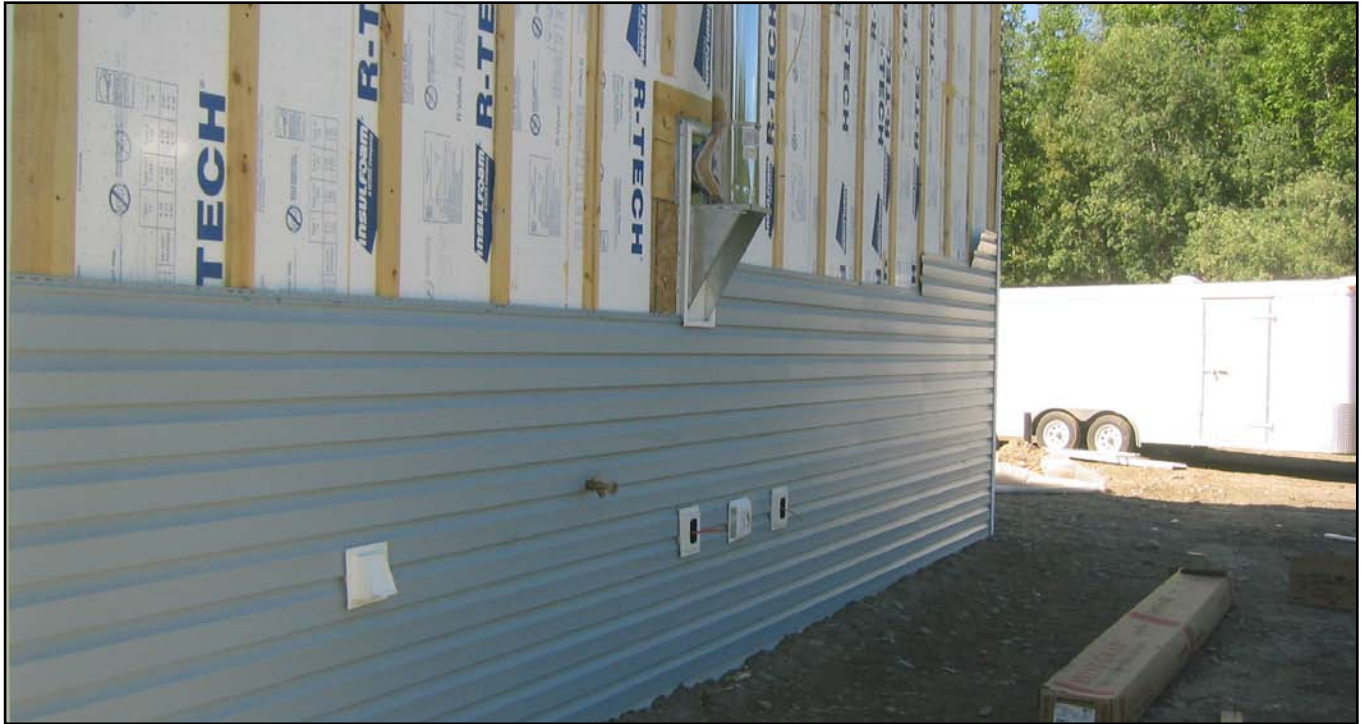
Image 32. Vinyl siding in progress, note furring around chimney support
