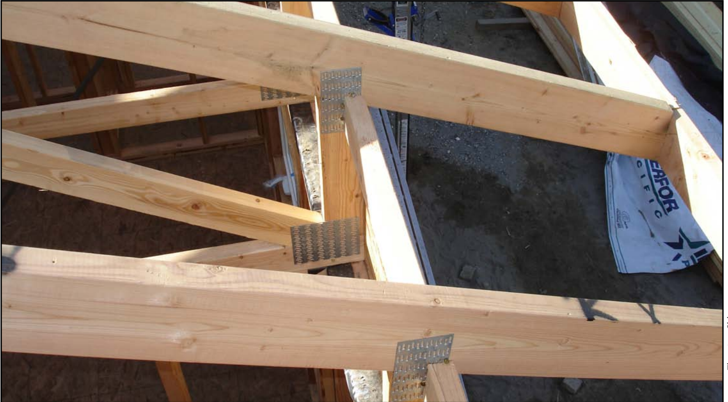
Image 1. Exterior View: 18-inch-deep energy heel truss allows for R-60 roof insulation and easy continuation of wall foam to the top of the attic insulation
