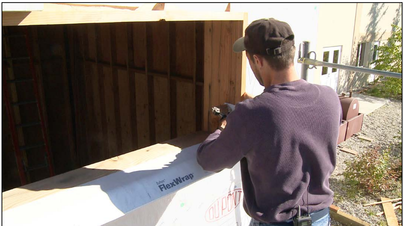
Image 9. Window buck sill detail with Tyvek® FlexWrap™
