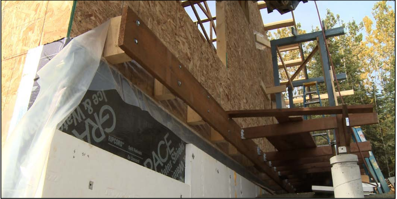
Image 6. Deck blocking and ledger board
