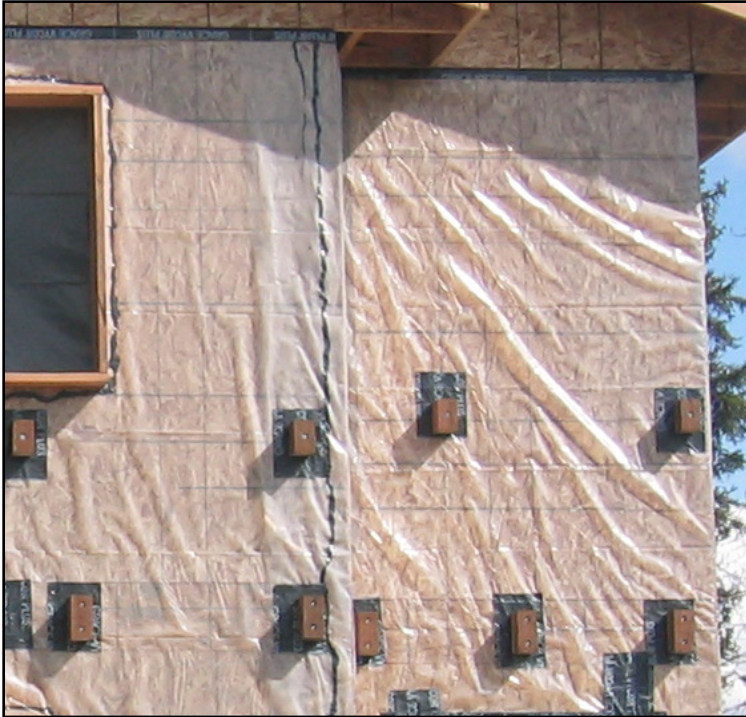
Image 3. Deck blocking over 6-mil polyethylene
