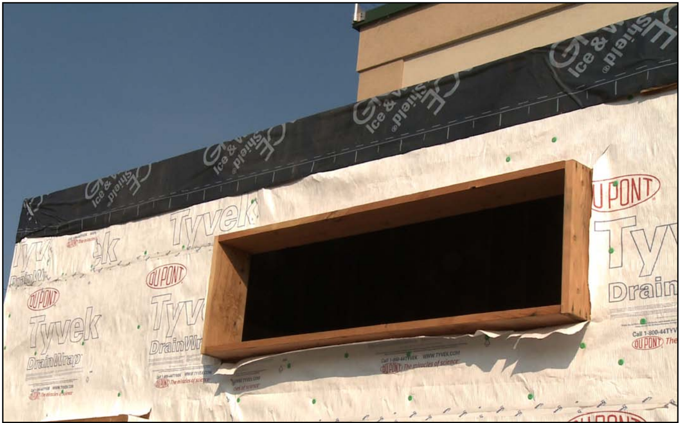
Image 8. Tyvek® DrainWrap™ is showing promise as an exterior membrane option, (as pictured here and the following pages on the CCHRC facility). It has met with code approval in areas of southeast Alaska, and its performance during sustained periods of extreme cold continues to be tested in Fairbanks.
