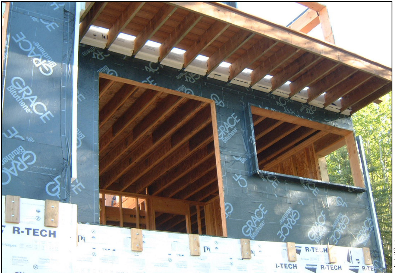
Image 5. Installed foam between cantilevered joists
