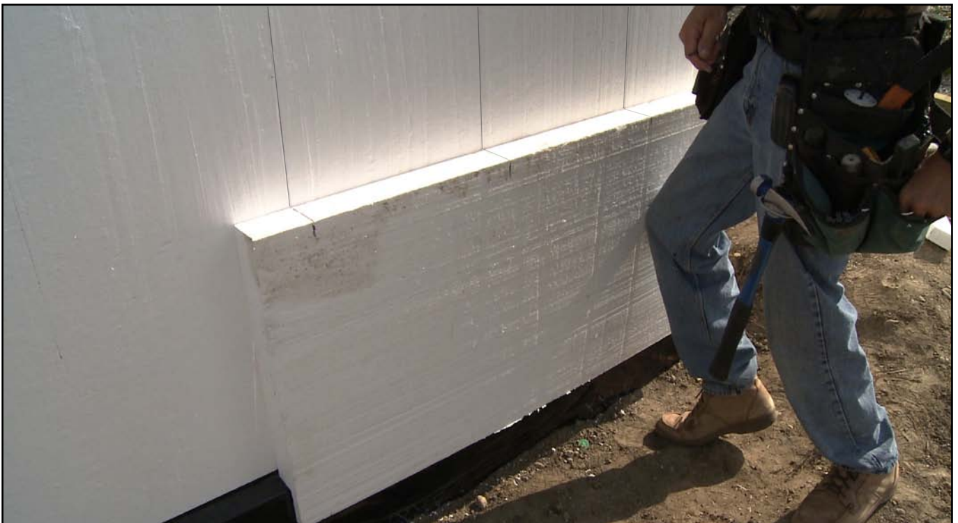
Image 26. Second layer of foam board is loosely attached using transferred stud pattern with eight inch screws and Wind-Lock® washers
