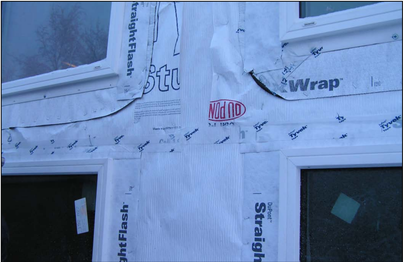
Image 17. Stucco preparation: Inset window flashing
