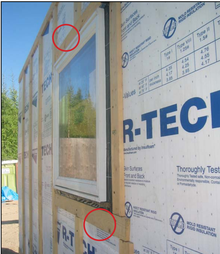
Image 33. Furring wraps around the window buck edges so the window can seal directly to the membrane on the buck. In wet climates, spaces above and below windows, and above doors, should be vented.
