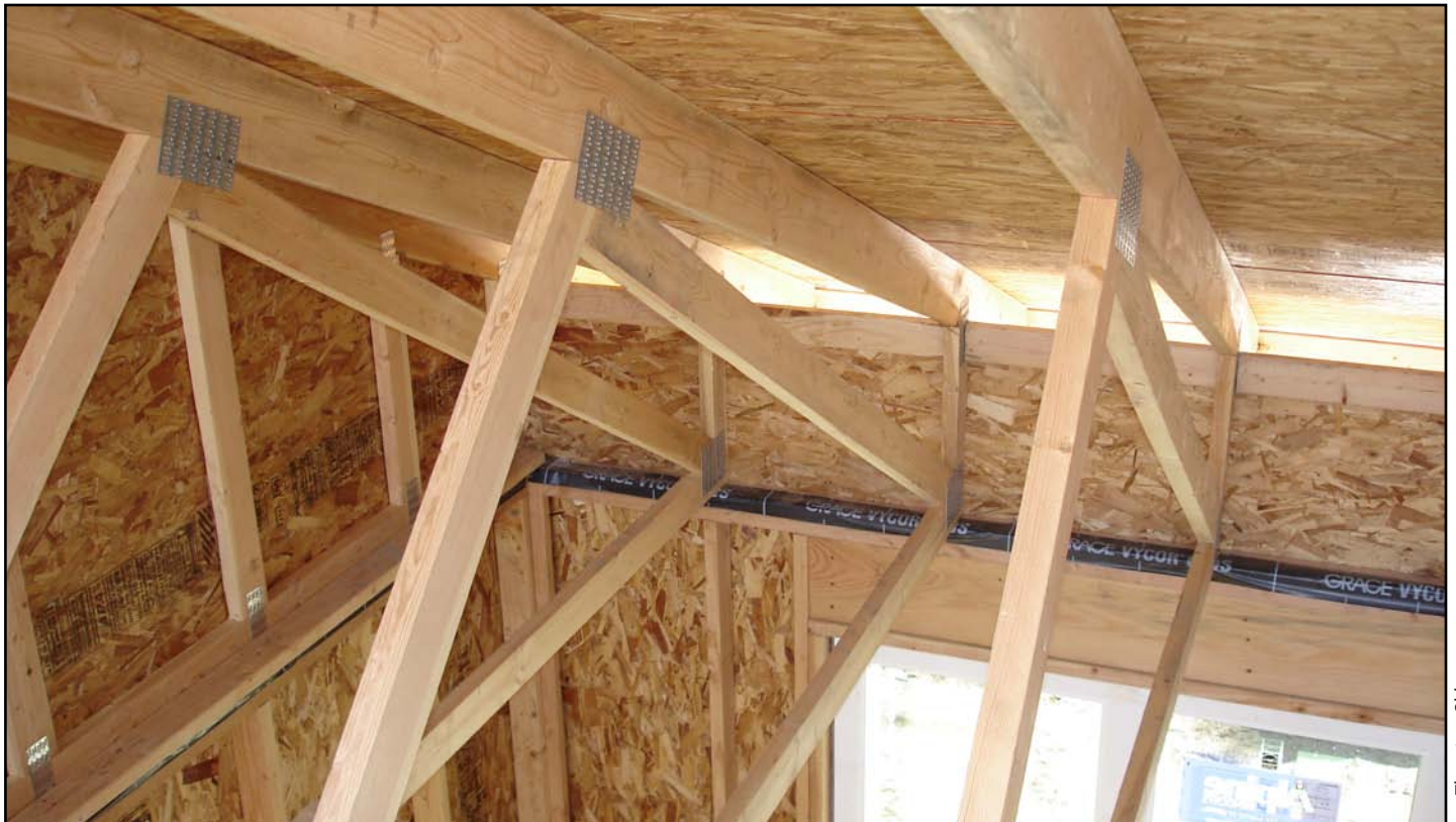
Image 2. Interior View: 18-inch-deep energy heel truss allows for R-60 roof insulation and easy continuation of wall foam to the top of the attic insulation
