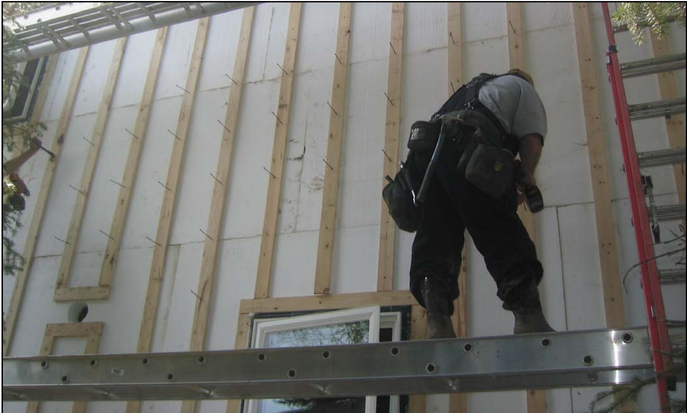
Image 30. Pre-drilled furring speeds installation process and keeps fasteners at a consistent height to avoid conflict with interior mechanical runs through the stud bays
