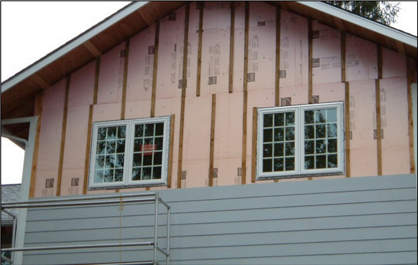
Image 35. Vinyl siding in progress. Note that all spaces between furring strips are vented rather than capped.
