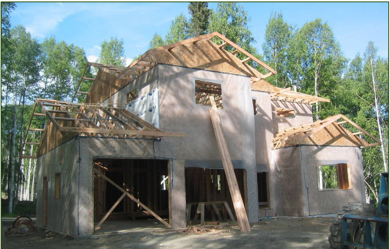
Image 20. 6-mil polyethylene exterior vapor retarder, note installation of foam board against wall before installation of garage gable truss. For structures outside of Interior Alaska, the exposed wall sections under the gable ends should have the exterior membrane extended to provide complete coverage.
