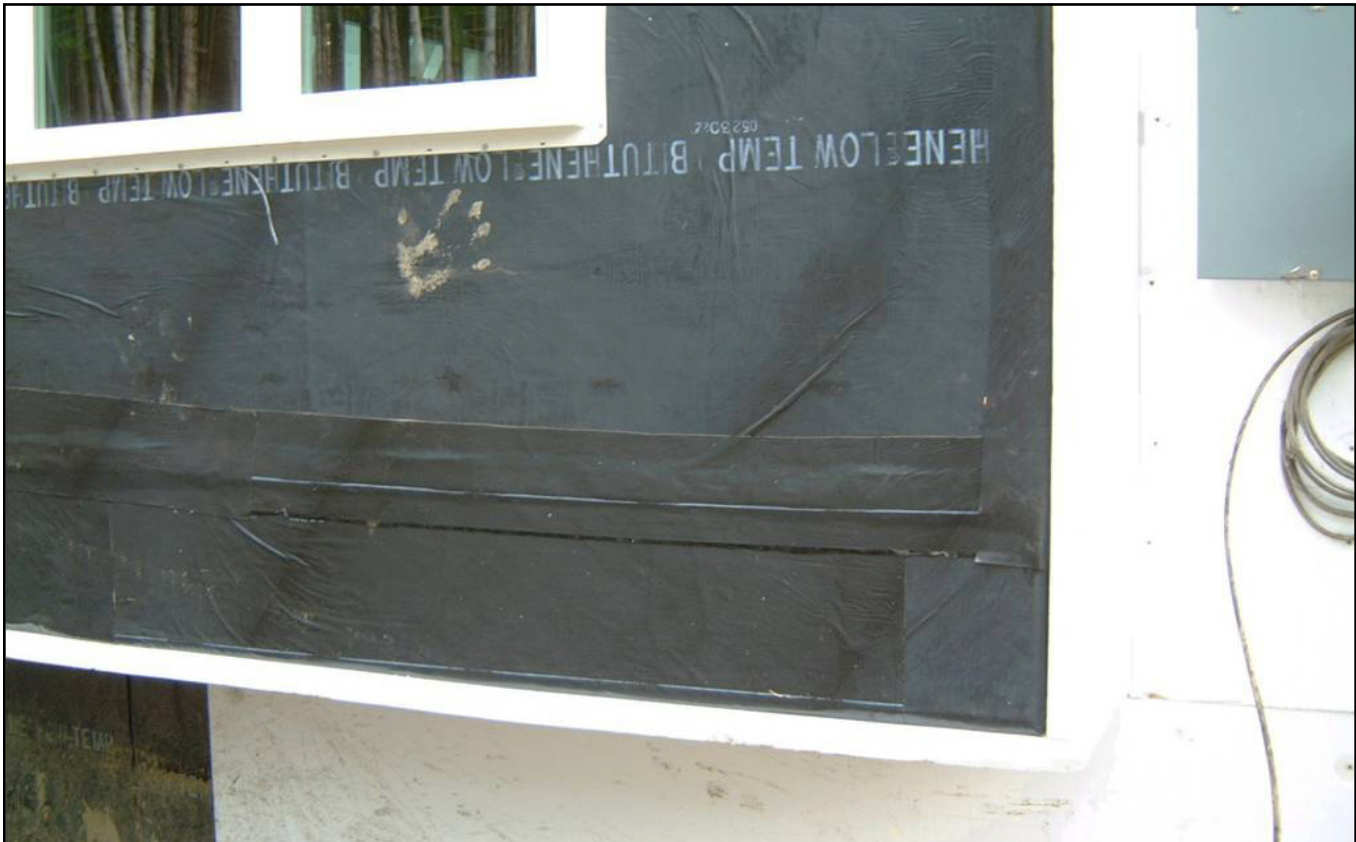
Image 27. Close-up of a square cantilever bay window with attached foam board
