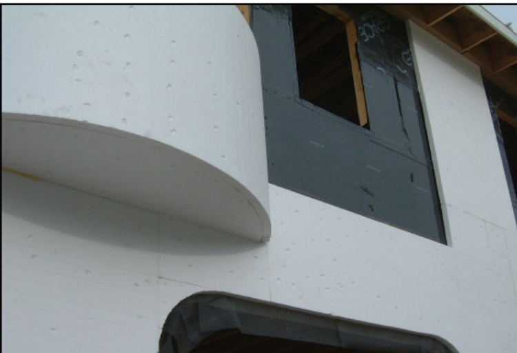
Image 28. Foam board covering a curved cantilever
