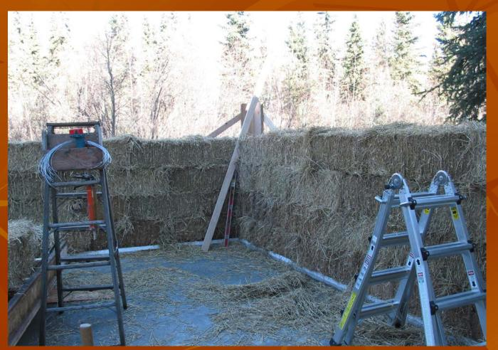
Jose sets the top plate and fastens the corners together. After the top plate is set the bales are preloaded using #9 wire run under the foundation and over the top plate.
