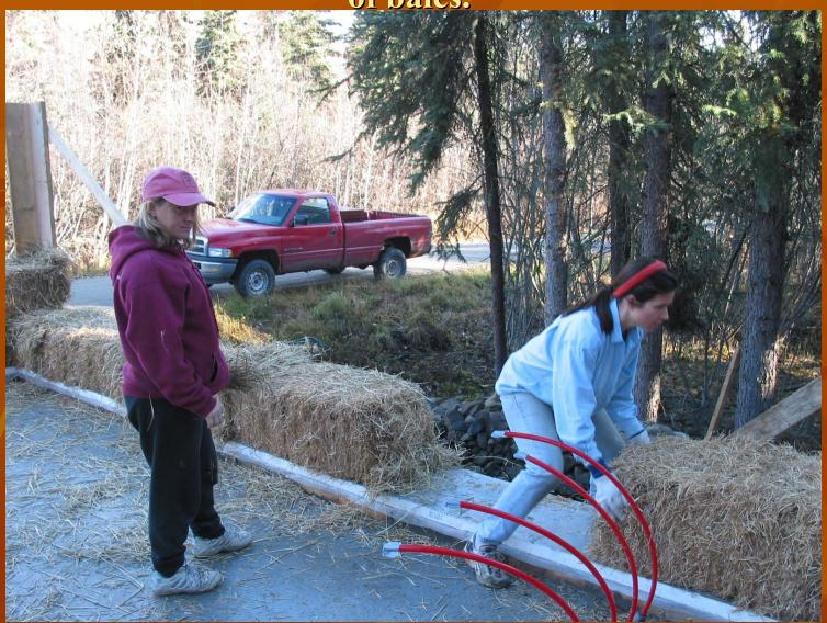
Four of the seven rows are finished at this point, and the wall is quite unstable. Once the wall is preloaded using the #9 wire and a special ratchet-like tool which is used to pull the wall down (preload), it becomes very stable.
