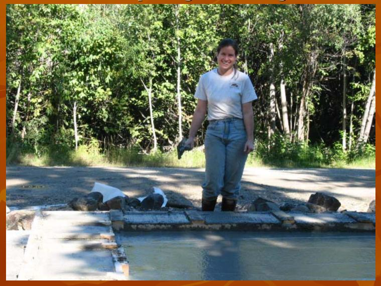
The floor and footers are poured with 2 x 4's inset into the concrete to use as nailers for the mesh lath around the perimeter. Note the foam on top which will act as a vapor retarder and capillary break.
