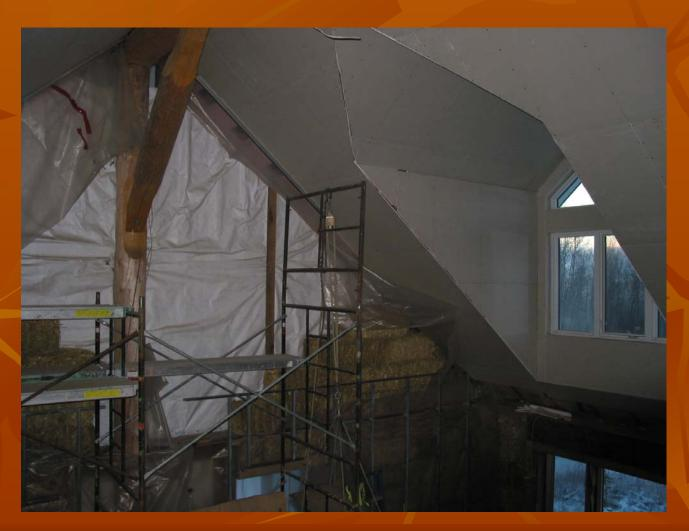
Straw is stacked in the north wall master bathroom. The 1 1/2" ledge allows for pouring the Gypcrete floor over radiant heating tubes.
