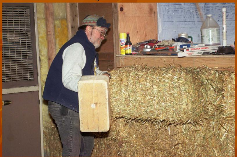
Straw is stacked in the master bedroom on the west wall. Notice the plywood ledge above the straw which is used as a fire block and helps to insulate between the "I" joist.
