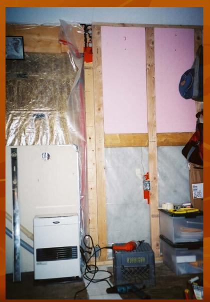
Some mold problems formed under the eves as the result of air leakage during the winter before the vapor retarder was installed.
