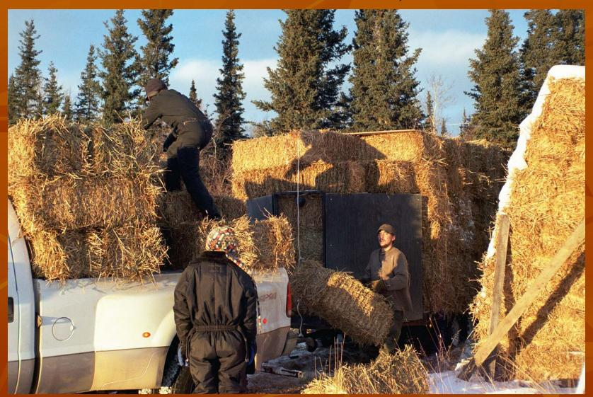
Gerald uses the Bonker to move the straw into place. It is best to trim and make adjustments when each bale is added.
