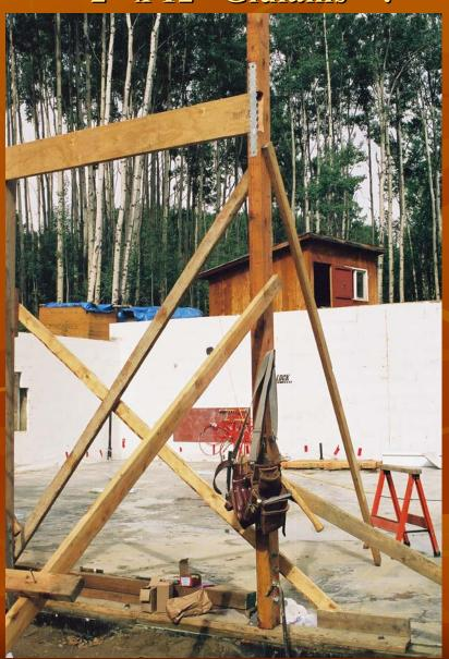
This shows the south wall in the basement. The west and north walls are from concrete filled foam forms. The framing is of 4" x 4"s and 2" x 12" Glulams ™. The slab contains hot water radiant heating tubes.
