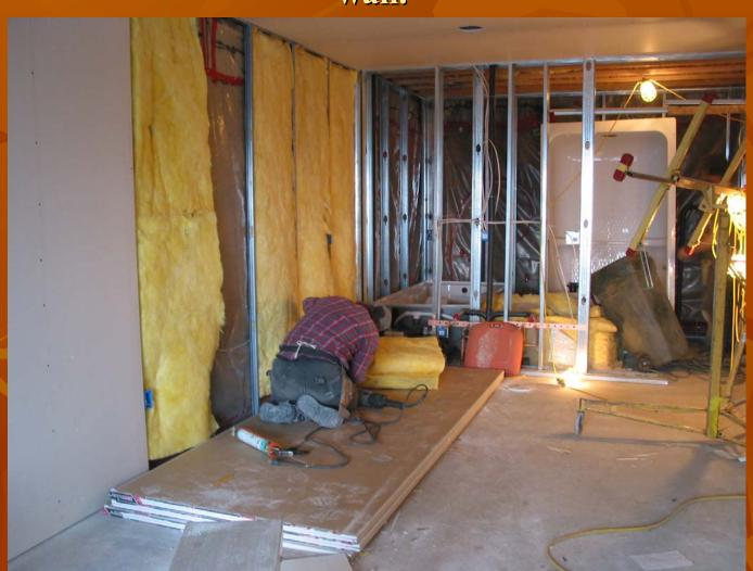
The east end is being sheet rocked. The alcove cavity was densely packed with cellulose after the rock was in place.
