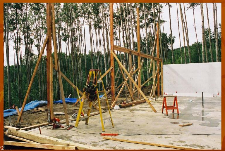
This framing is in the north wall on the first floor. Notice the Simpson ties and strapping. The west roof support post is being raised
