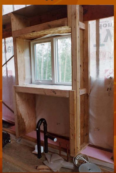
The gap between the 1 5/8" studs and the vapor retarder is filled with sound bats to eliminate convection loops in the wall.
