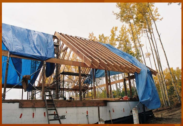
Closed in for the winter, the South face is sheeted with plywood for shear strength because of the many openings for windows and for the large 8' patio doors. Straw was stacked all during the winter.
