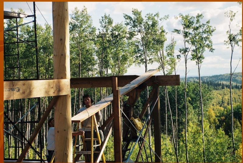
The east post is set into the cradle made of Simpson #10's bolted through 12" x 12" Glulams tm with 7/8" diameter bolts.
