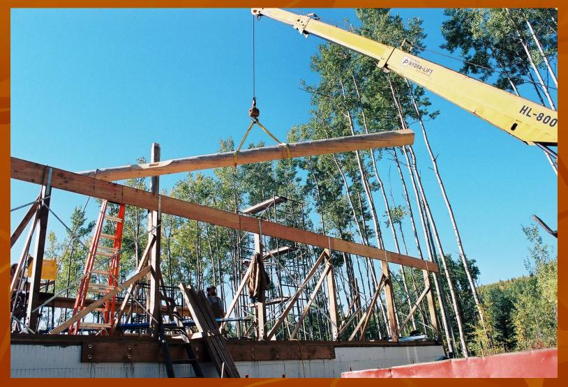
The 52' ridge pole is lowered into place. Notice the mortise and tenon joints.
