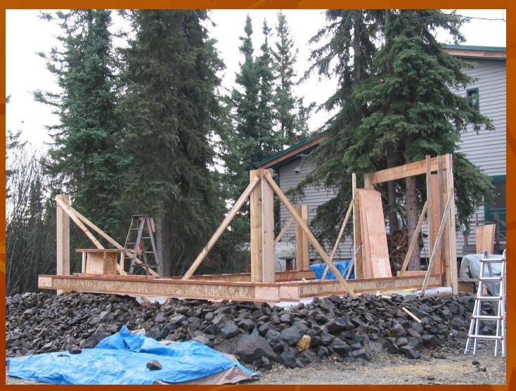
The "I" beam top roof plate assembly is ready to place as soon as the bales are stacked.
