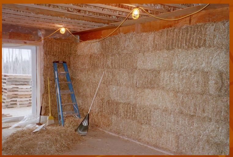
This shows detail in the ceiling. There is 12" (R-38) fiberglass between the webs, then 1" foam is placed between the flanges. Mathew is stuffing straw into the triangular space formed at the junction of the roof and straw.
