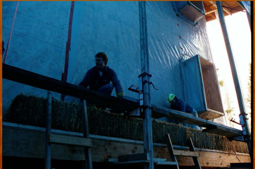
Bales are stacked around the window bucks. The rebar is driven through 1 1/2 bales, and then wire is run through the acoustic screw and wrapped around it which holds the bales tightly against the wall.
