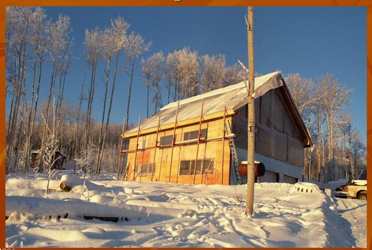
Steel hat channel is run vertically for attaching the siding to the wall with Tyvek underneath. The garage wall is a 2" x 6" framed wall with 2" of blue foam on the outside.
