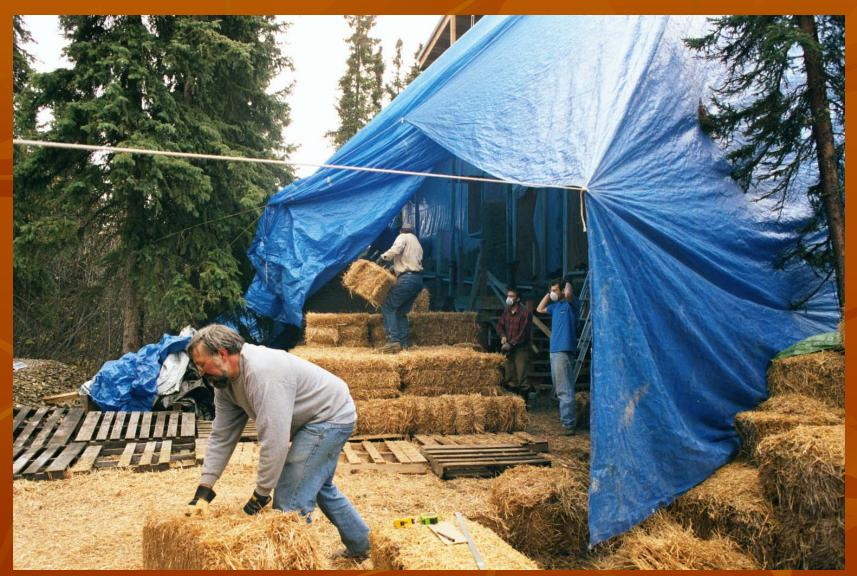
The first row of bales is laid on the ledge. Notice the vapor retarder on the outside and the window openings.
