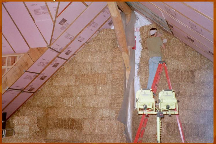
Bales are stacked for the 21' east wall using scaffolding and a block and tackle. Notice the visqueen tabs which are part of the continuous air/vapor retarder system.
