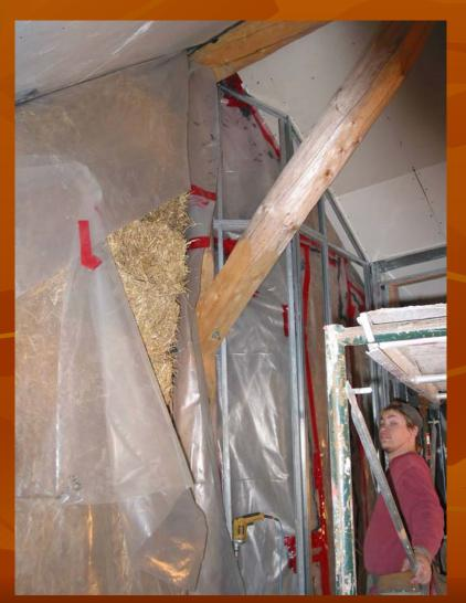
The "window bucks", as they are called in the straw bale community, are being framed. The cavity is filled with straw and capped with OSB. The ledge on top of the Glulam™ was also filled with cellulose.
