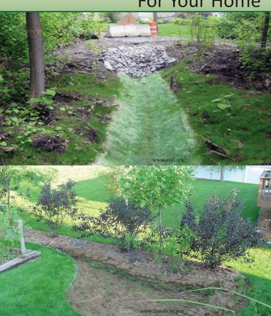
A vegetated swale is usually a grass-lined depression. Plants slow down runoff water velocity and infiltrate the water into the soil. Swales can be used to redirect rainwater runoff to rain gardens, tree pits, and dry wells.
